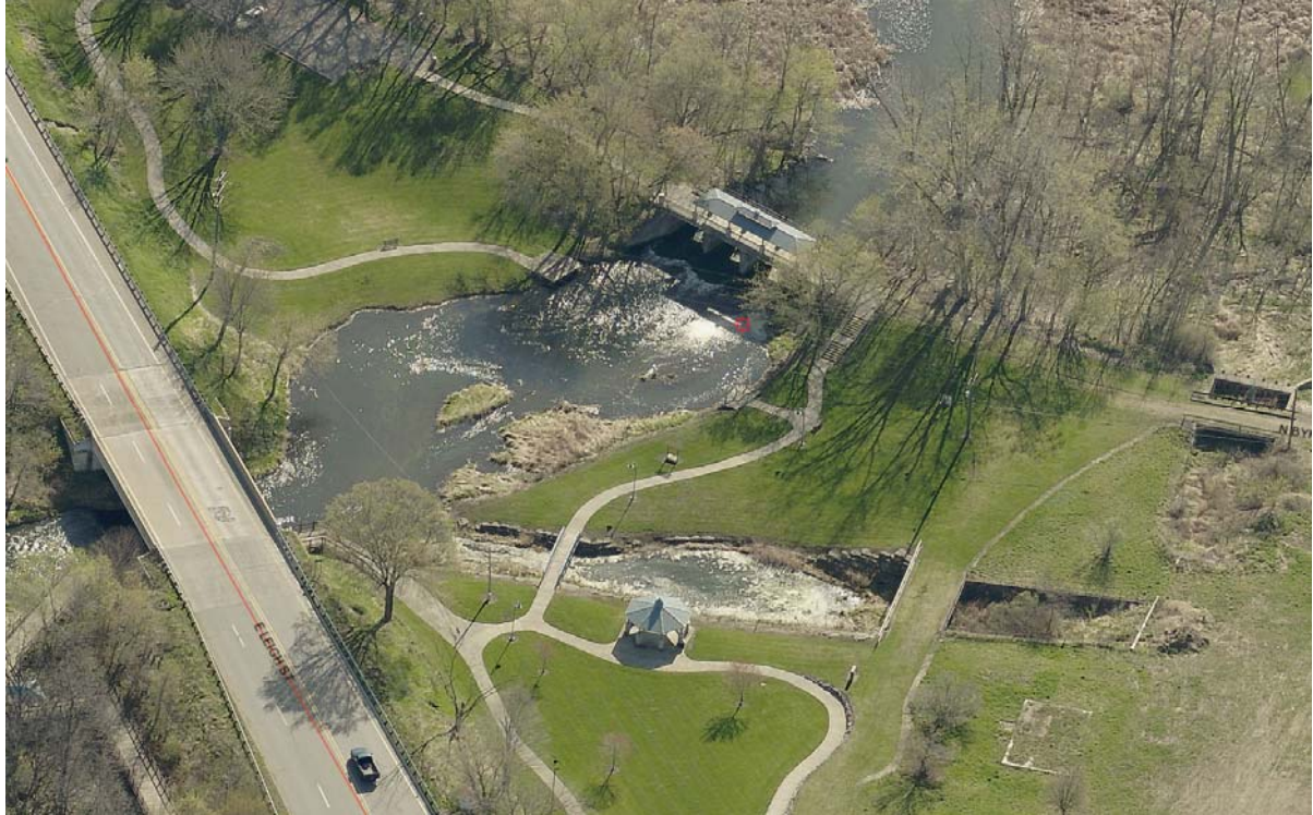
Homer's former Mill Pond Dam (for the grist mill)
